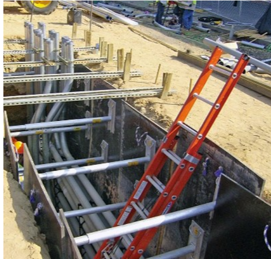
[Mock picture of proper set up of a ladder in a trench]
