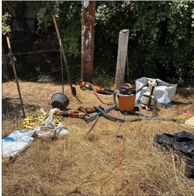
Excavation site with dry vegetation
