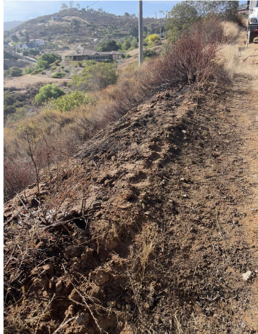
Area where fire occurred during annual grading operations
